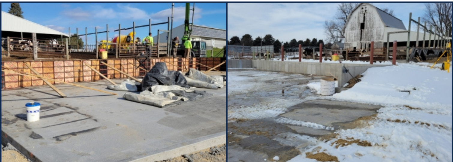
Project progress during and after construction of the manure slab on the Timms' farm. Photos by Winona County SWCD.
