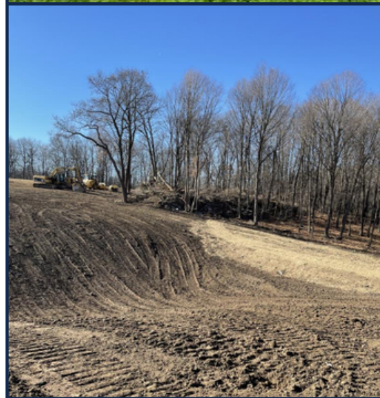
Images during and after the installation of a grade stabilization structure in Whitewater. Photo by Winona County SWCD.
