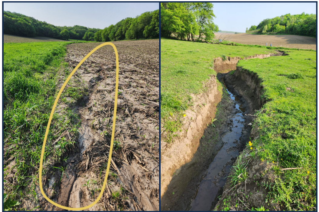
Diverted water (circled in yellow) along the grassed waterway (left) and pasture gully (right) before reconstruction. Photos by Olmsted SWCD.
