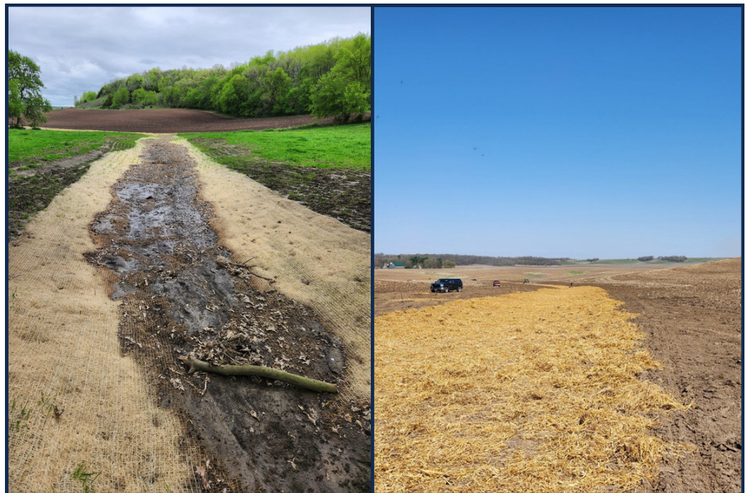
Filled pasture gully with erosion control (left) and reconstructed grassed waterway during seed establishment (right). Photos by Olmsted SWCD.
