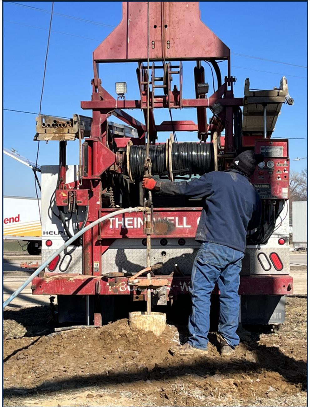
Contractor preparing to seal the Altura Well. Photo by Sheila Harmes.
